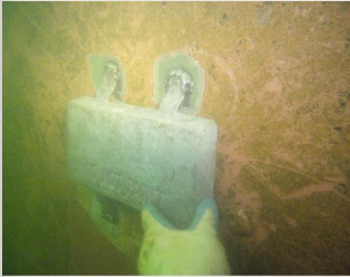
ANODE INSTALLED FROM PAGE 1 STORY
